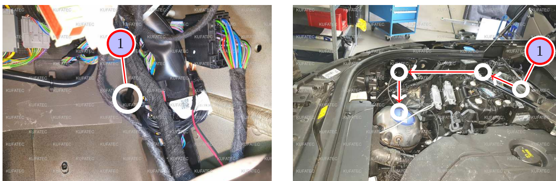
Figure 11: Cable routing to the front sound generator
